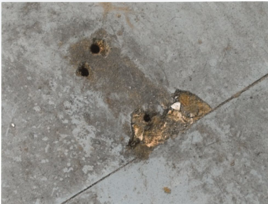
Photo 25: The mounting place had more than a pair of mounting holes.
