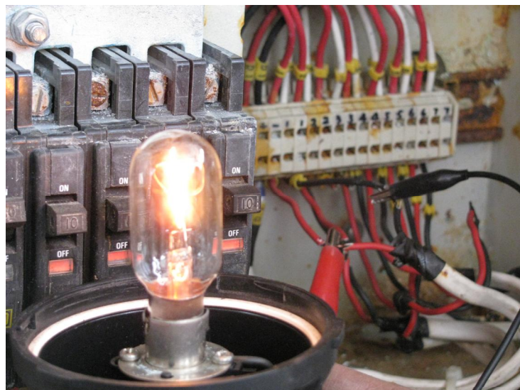
Photo 13 The insulation of wires in Circuit 2 was stripped to allow the connection of the 12 V power supply to the test circuit. Upon connecting the Test Light Bulb to the Port Light circuit, the Test Light Bulb lit up to confirm positively that this circuit is the circuit for the Port Light.
