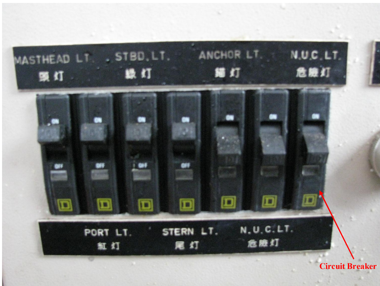
Photo 2 Circuit Breakers controlling the various lighting circuits
