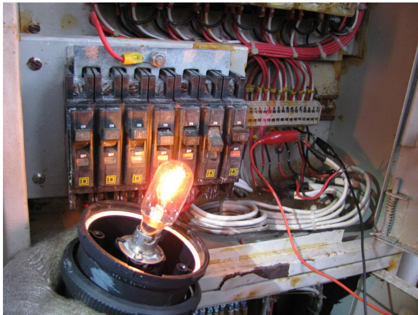
Photo 15 The insulation of wires in Circuit 4 was stripped to allow the connection of the 12 V power supply to the test circuit. Upon connecting the Test Light Bulb to the Anchor Light circuit, the Test Light Bulb lit up to confirm positively that this circuit is the circuit for the Anchor Light.
