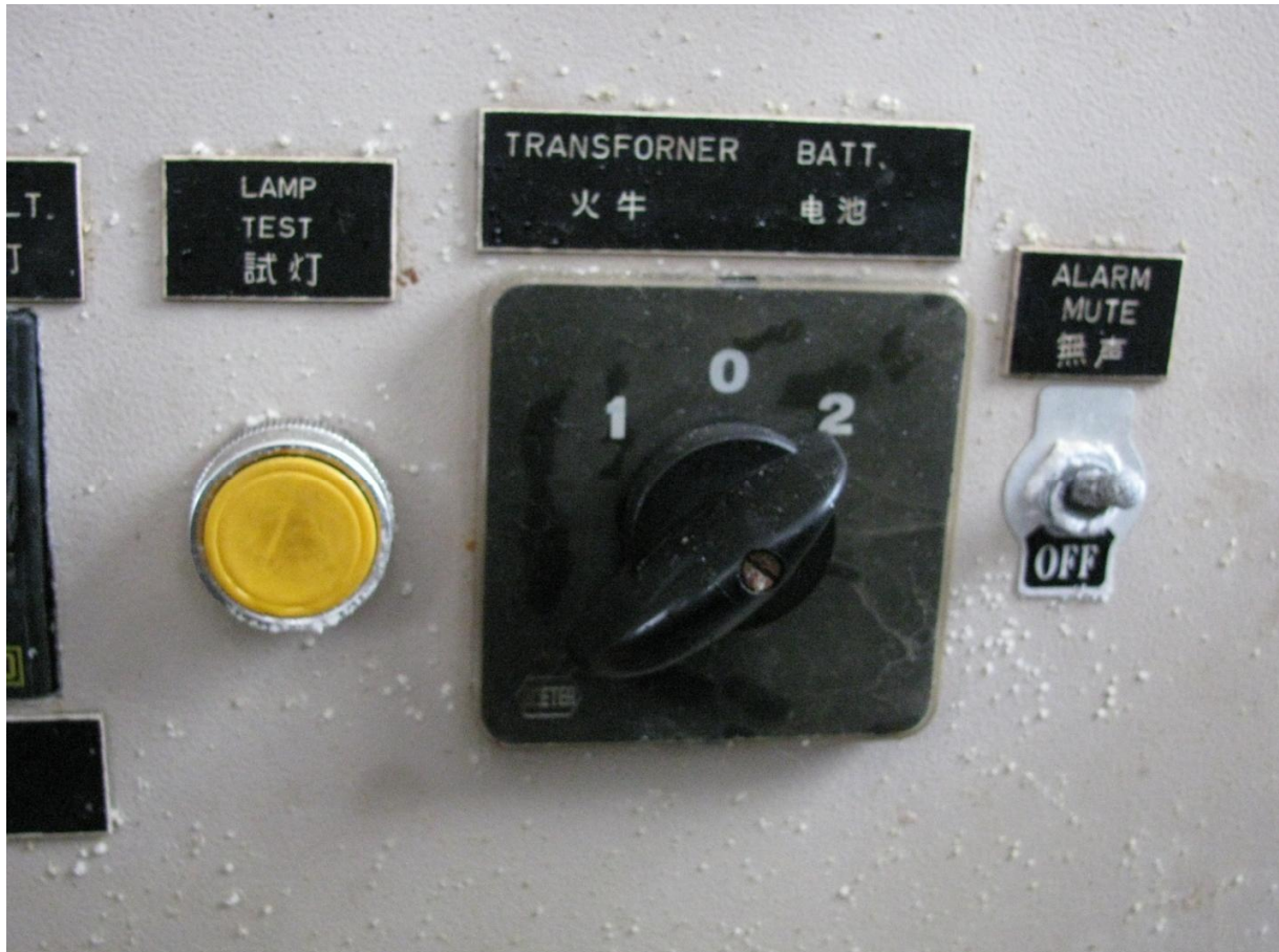
Photo 1 Power to the various light circuits can be obtained either from the Generator or from the Batteries Pack. There should be no differences in the functionality of the circuits no matter where the supply was derived. However the power from the generator would be more stressful to the components (such as lamps) if the voltage rises above a certain threshold value. For example, if a 24 V lamp is fed from a 26 V source, there is more power pumped into the lamps, thereby shortening the life expectancy of the lamps.
